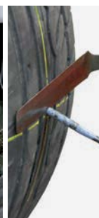
8 Seal the MINICOMBI base and any still exposed buffed areas with INNERLINER SEALER and cut the stem.
