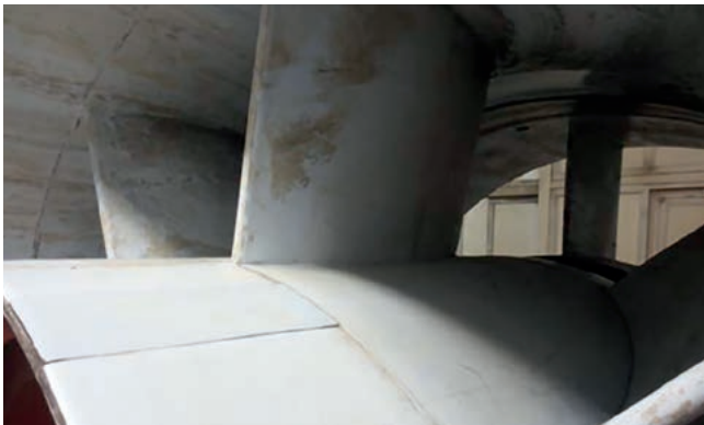
REMAFLON as non-stick lining in a flue gas ventilator
