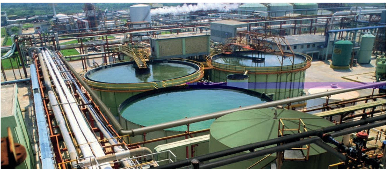
Rubber-lined sedimentation tank
