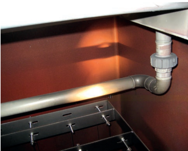
COROFLAKE coating in a wet ESP
