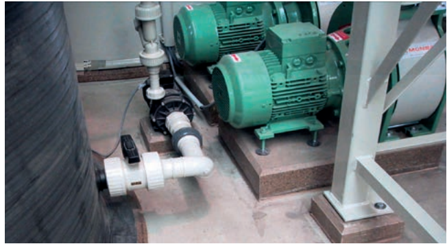
Polly-concrete bricks as pumping equipment foundation
