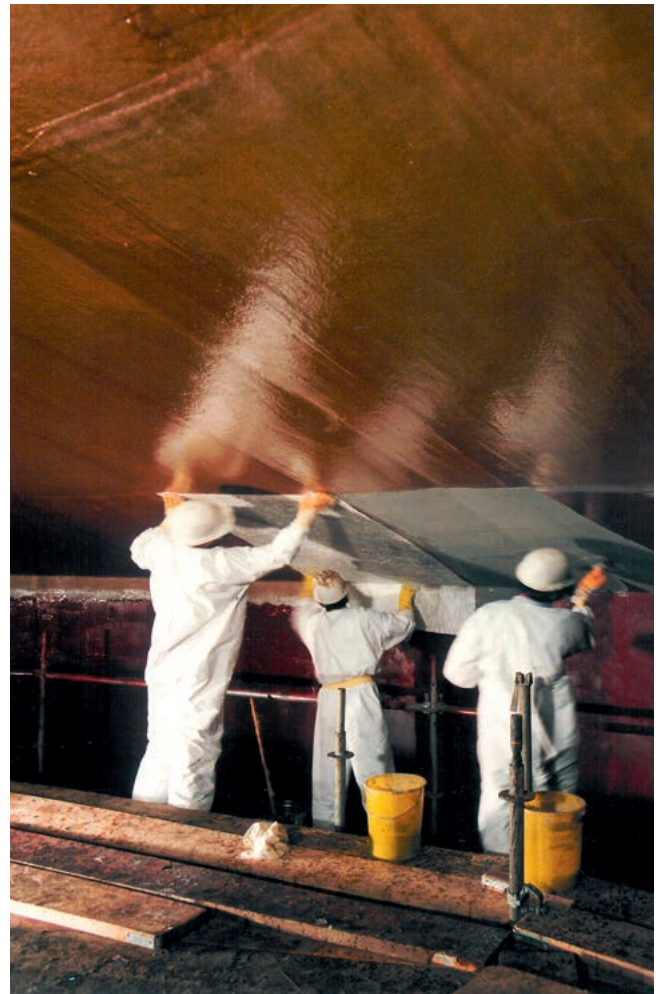
Installing a laminate coating
