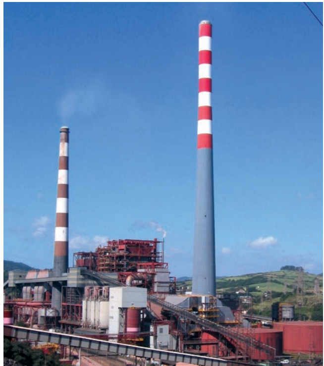
Coated power station chimney
