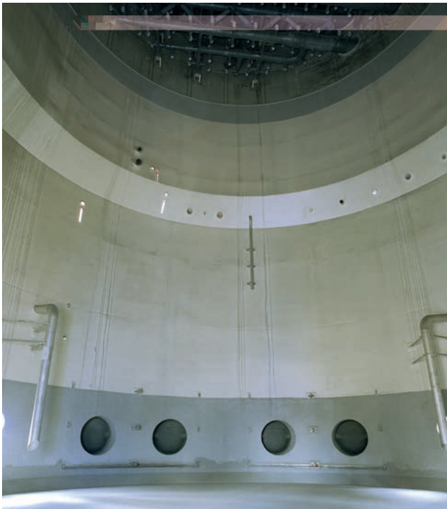
Lined flue gas scrubber
