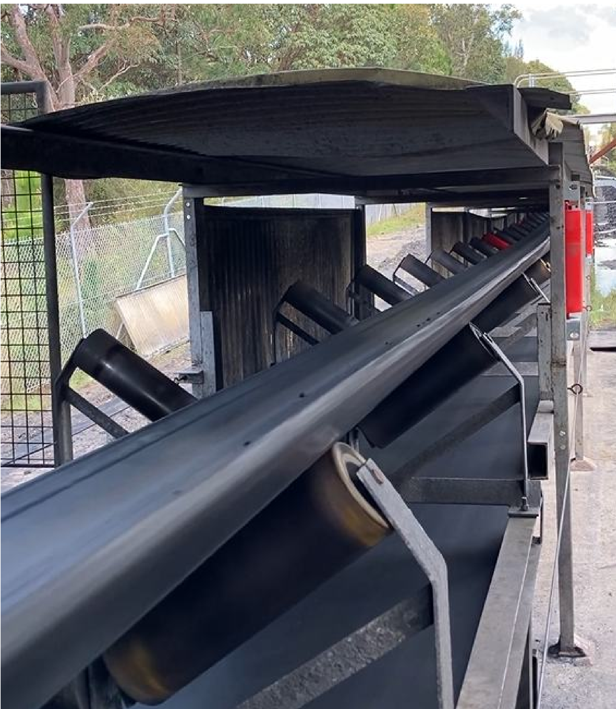
Tracking before installation of REMATRACK TTX
